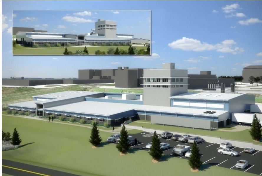
P068 Electromagnetic Sensor Facility
