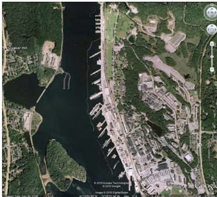
ST09-0339 Waterfront Repairs
