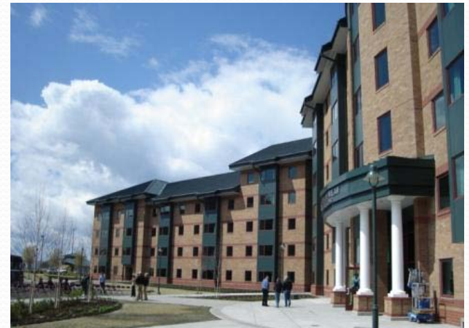
BEQ, NS Everett, WA – LEED Gold
