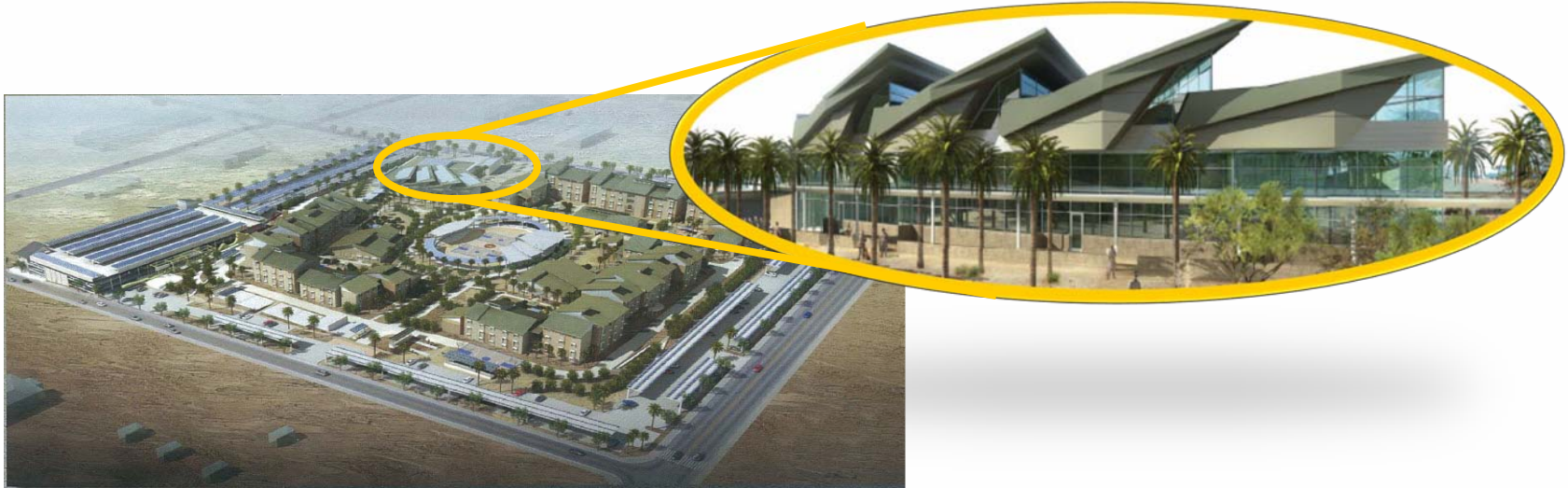
North Mainside Area including P163 BEQ & Parking (MCAGCC 29 Palms)
