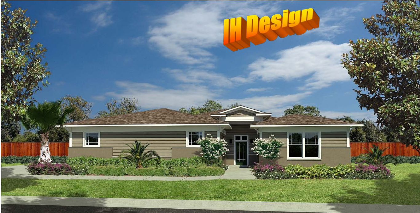
Replace Base Housing, GTMO
